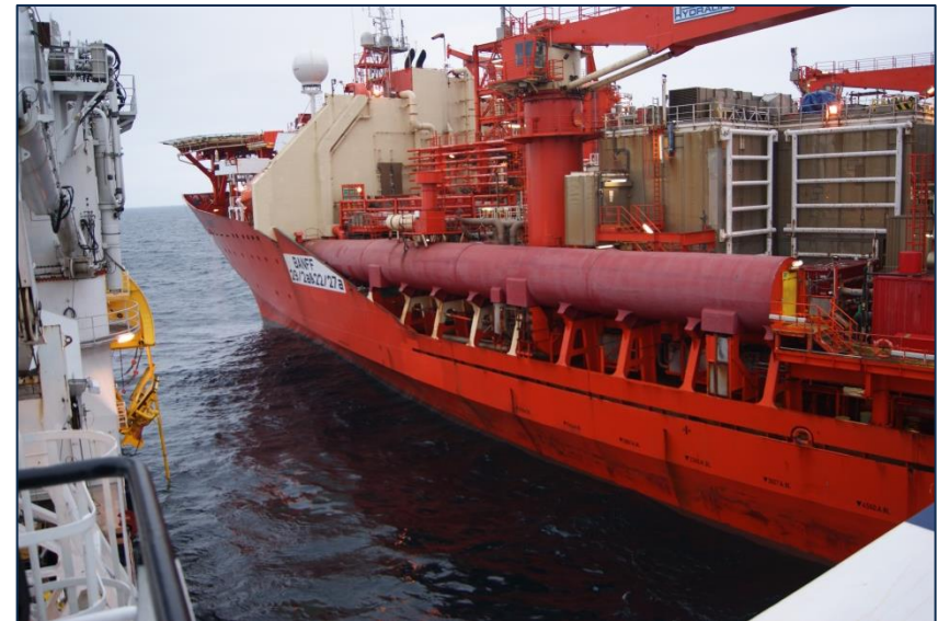
Banff FPSO on the Banff Field in May 2014
